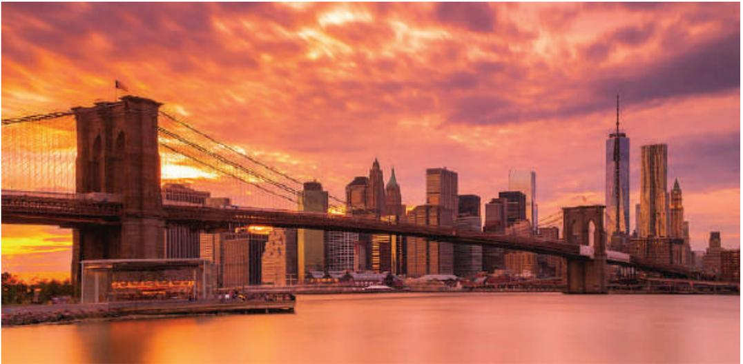
19th century and remains one of New York's most popular and well known landmarks. The impressive bridge spans the East river between Brooklyn and Manhattan and stretches for a length of 5989 ft, about 1.8 km. The span between the large towers measures 1595.5 ft (486 meters). This made the Brooklyn Bridge the world's largest suspension bridge.
